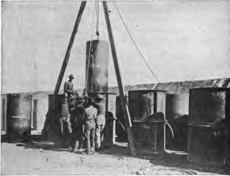
FIG. 160.—Removing Inside Steel Forms from Concrete Pressure Pipe, Boise Project.
